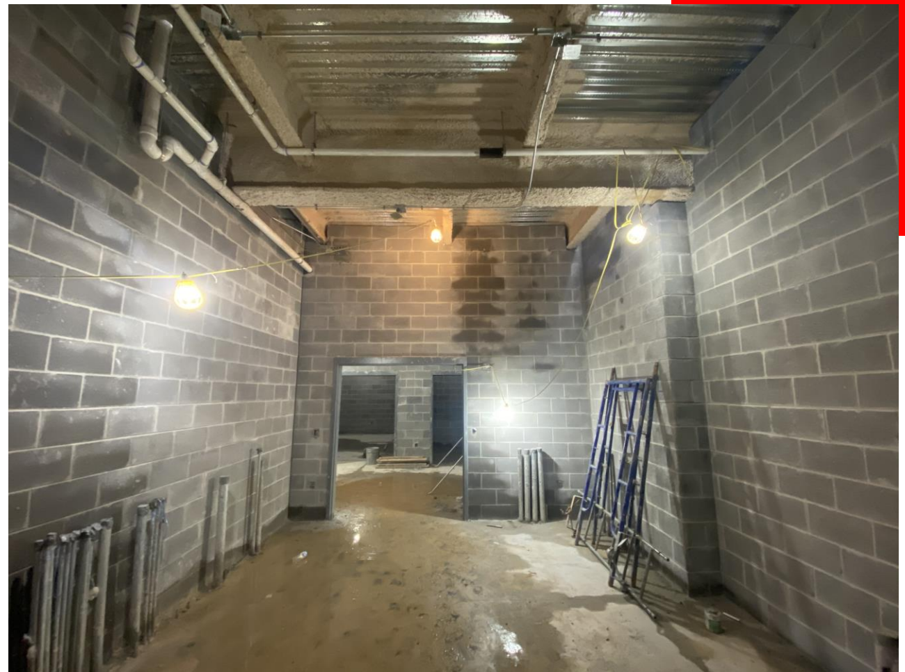
1 st Floor of New Addition CMU walls complete
