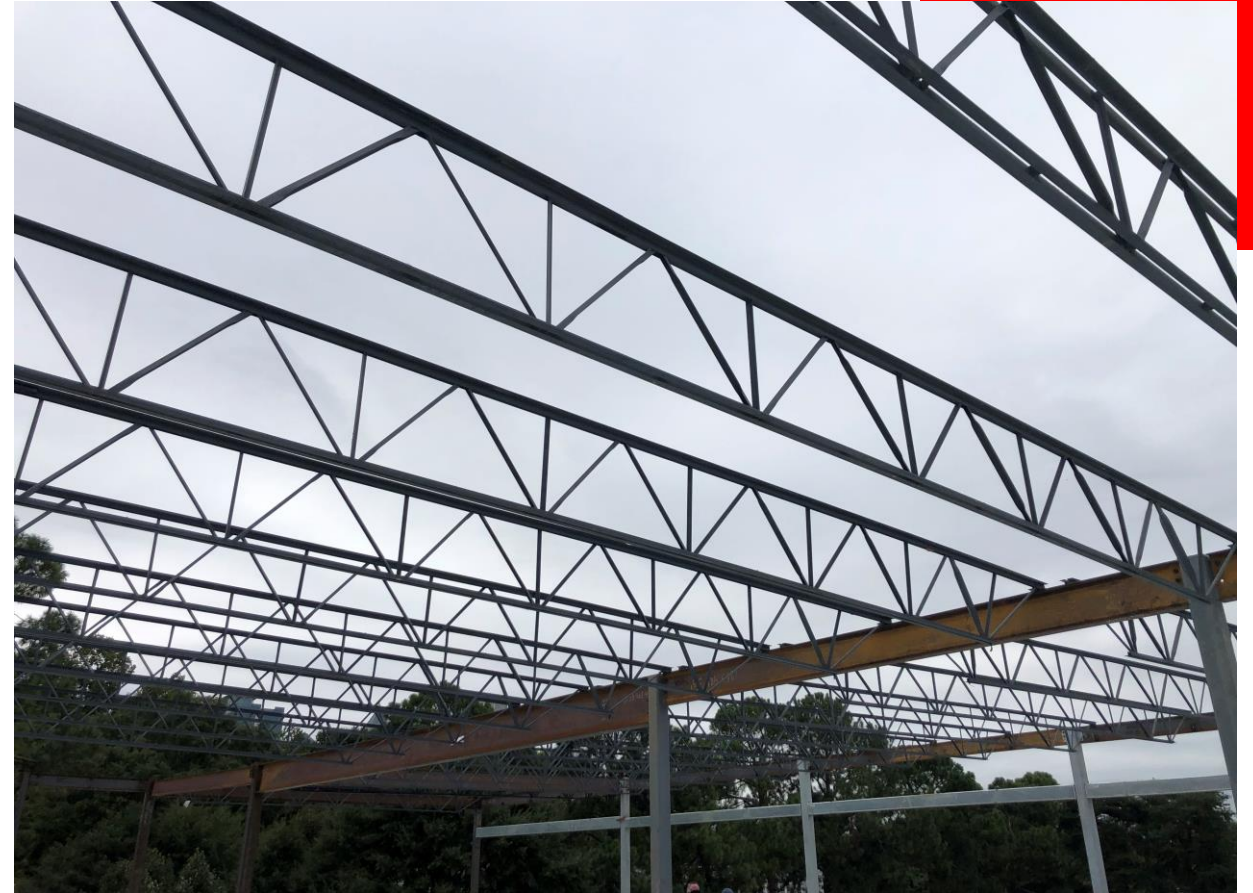
Bar Joists installed at New Addition Roof
