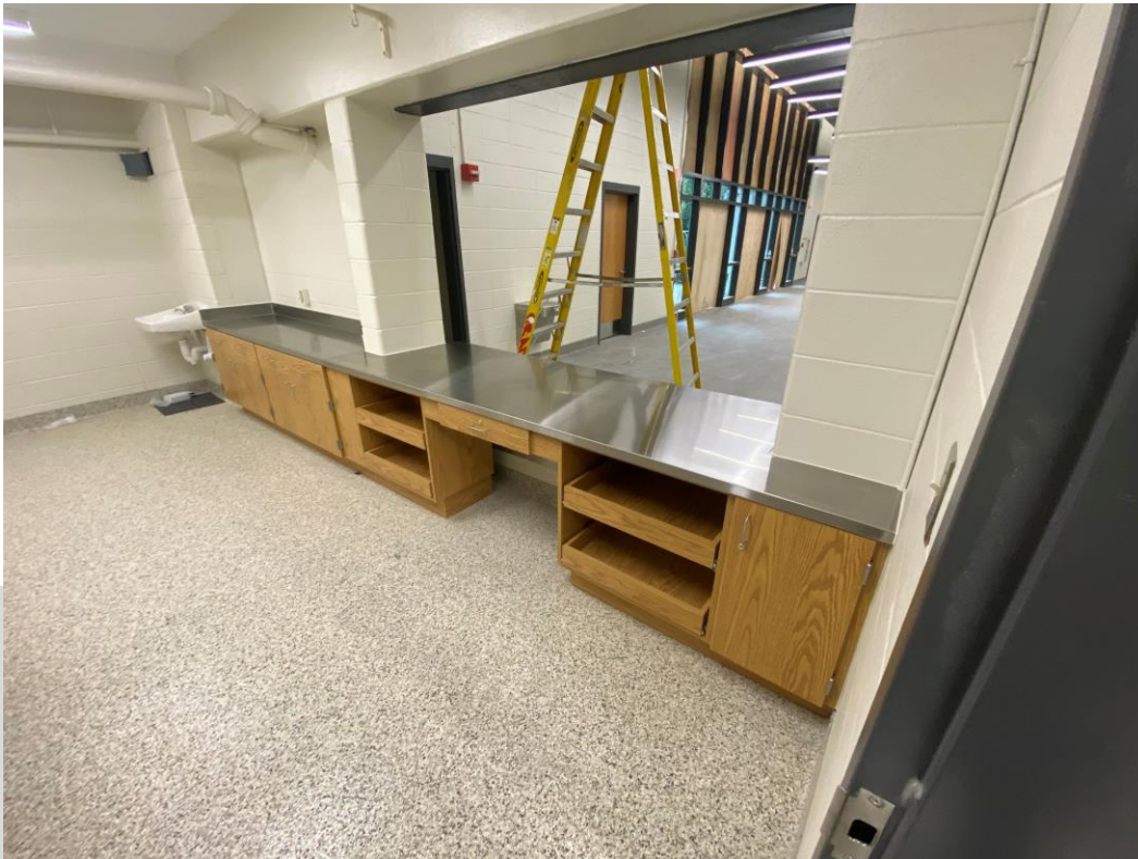
Casework and Stainless Countertop installed at the Performance Gym Concession Stand
