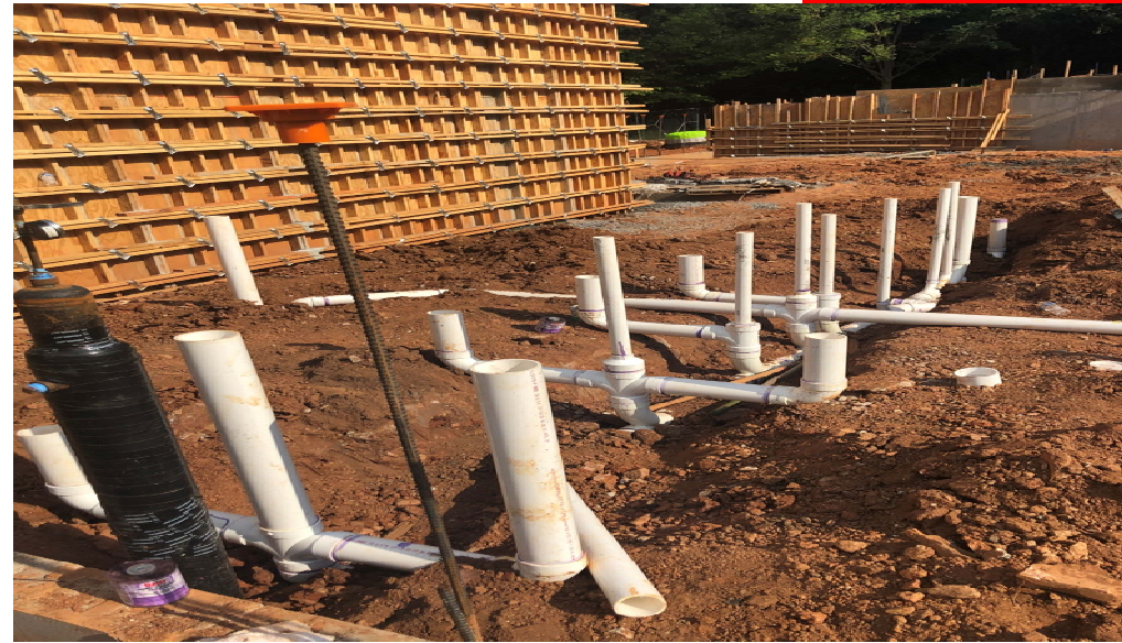
Underground Plumbing for new addition
