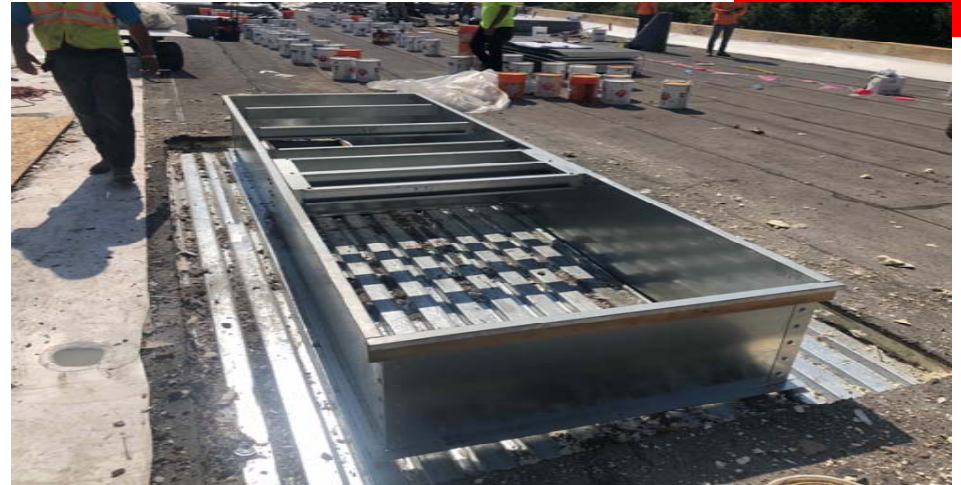
Installing HVAC Curbs on 8 th Street building
