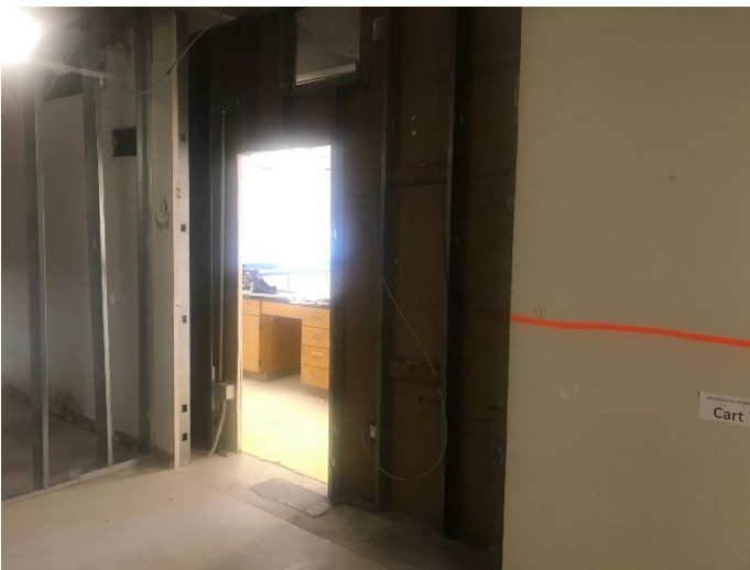
Picture 7: New door openings in Area B
