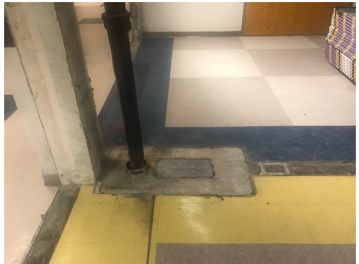
Picture 4: Concrete patching for existing chases
