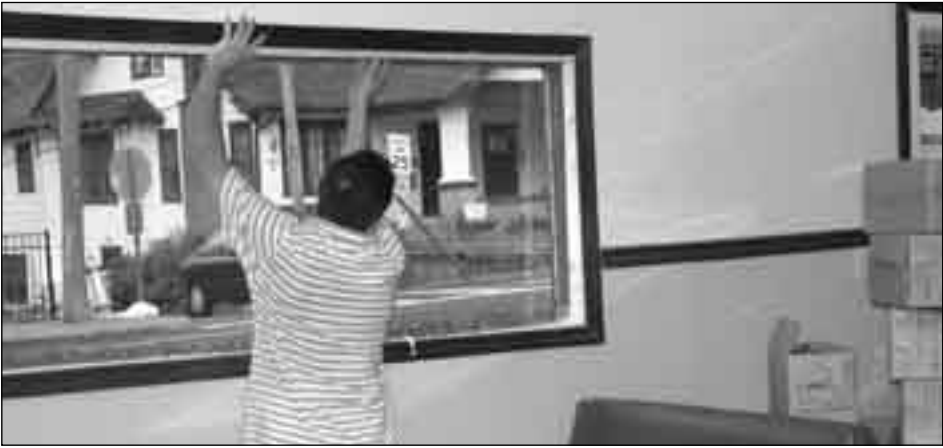
SILVER LINING: A construction worker measures the length of one of the Silver Grill’s windows. Almost 10 months after closing, the Southern-style restaurant is reopening its doors for business under new ownership.
